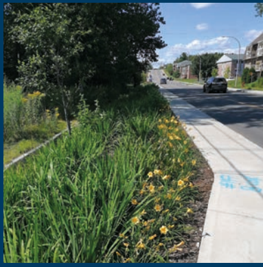
Group of bioretention filter systems for stormwater treatment located on Saint-Maurice Street in Trois-Rivières, Québec.
